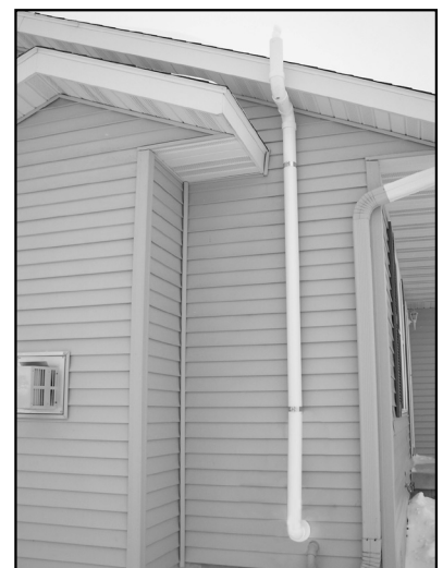
Figure 12 Vent Line Installation (3 inch)
